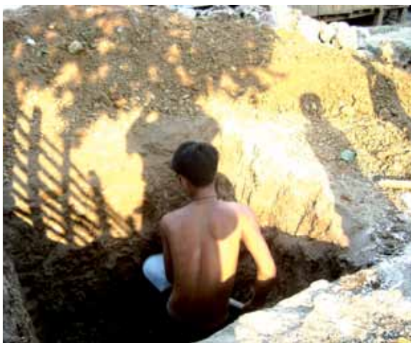
Digging latrine as part of community sanitation program in Karenni State
